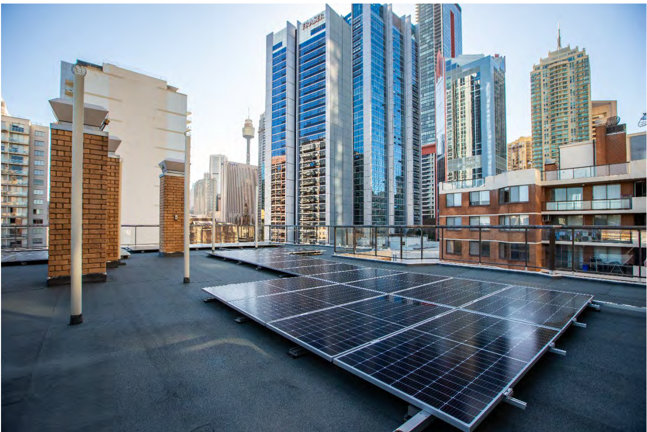
Image 7. Solar panels on the rooftop of the Windsor Plaza apartment building in Sydney city centre. Photo by Katherine Griffiths / City of Sydney
